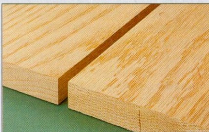
CURVED GRAIN. To avoid drawing attention to a joint line, arrange boards so curved patterns merge.
